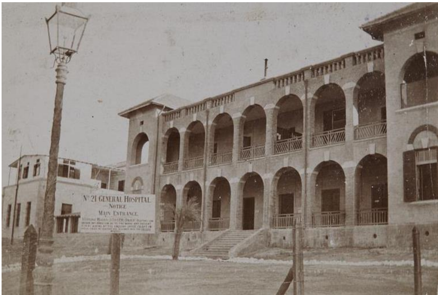
General Hospital at Ras-el-Tin, Ghezireh
