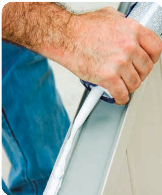
Caulking around window frames.
