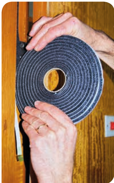
Fitting a weather strip to a door frame.
