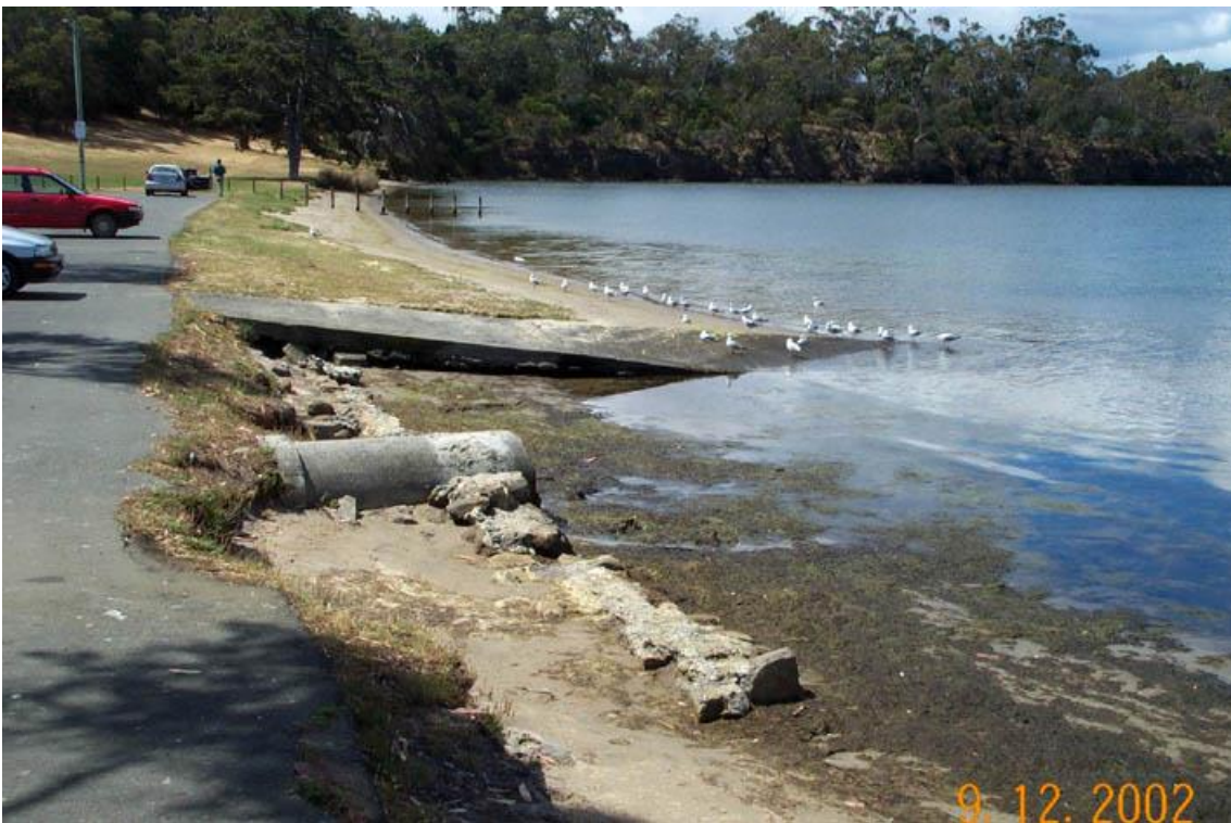
Figure 20: A non-resilient artificial shore. This short stretch of inadequate ‘armoured’ shoreline at Cornelian Bay in 2002 had failed to perform properly and was backed by an erosion scarp progressing landwards behind it! However because of a commitment to protect the shore, this under-performing artificial shoreline was later replaced with the much more resilient artificial shore shown in Figure 19 above. Photo by C. Sharples (2002).
