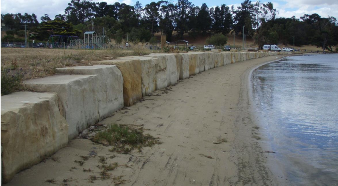
Figure 19: A resilient artificial shoreline at Cornelian Bay, Hobart. This coastal open space is a highly valued asset in Hobart and thus the artificial shoreline seen here can be expected to be maintained. This is demonstrated by the fact that this robust coastal protection structure was constructed to stop relatively rapid erosion of this shoreline, and in part replaced an earlier coastal protection structure that was failing (see Figure 20). Photo by C. Sharples (2013).
