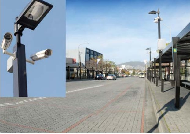
The new CCTV monitoring system at the Rosny bus mall.
