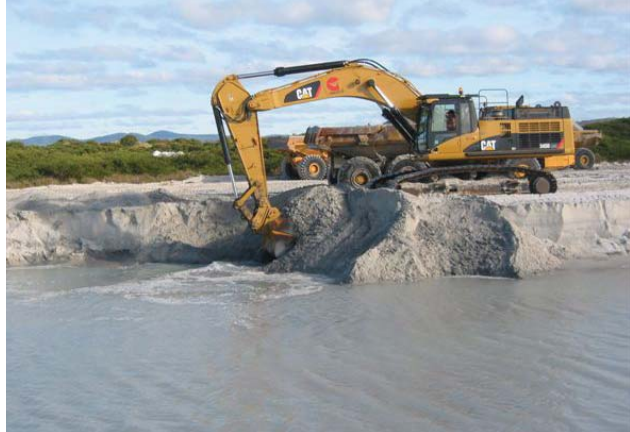
Works commence on the removal of sand to improve access to the port of St Helens.
